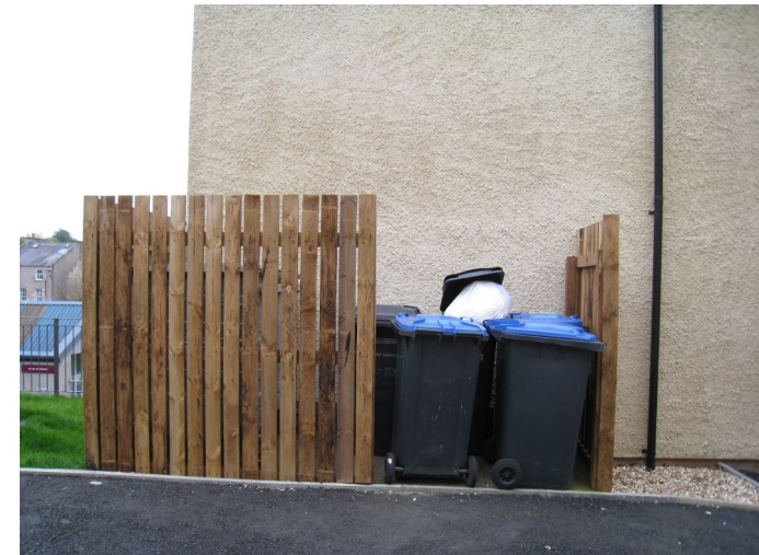
Example of bin storage area which is too small, not allowing sufficient space for filling and emptying bins
